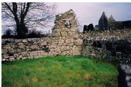
Structural remains of St Colman's Oratory
